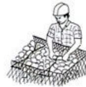
At the time of erection large numbers of boxes/mattresses are used - it is necessary to tie and so as to form one intergrated structure. Tie wires are selvedge wires of adjoining Gabions at regular intervals. secured by triple loops.
